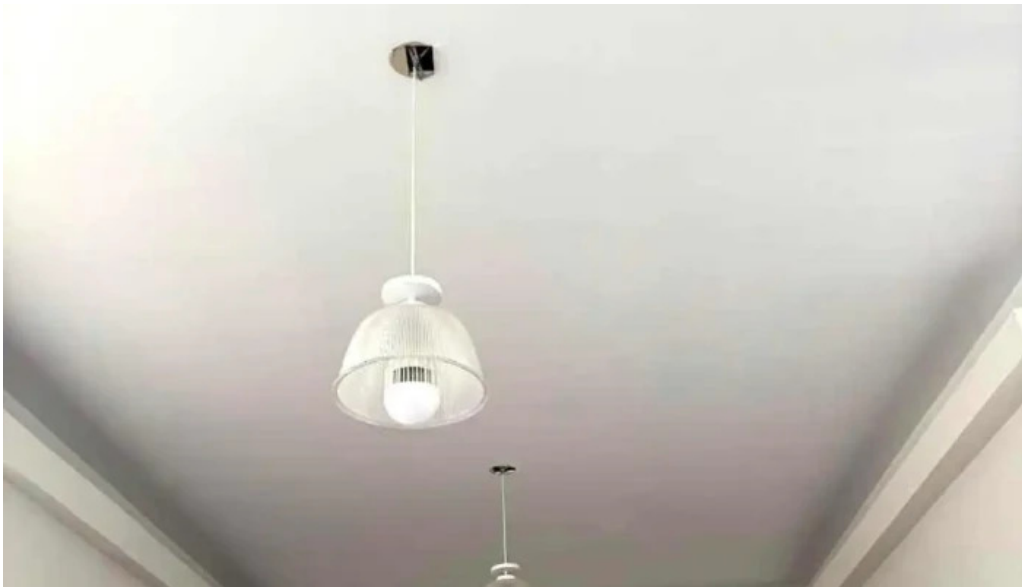
Electricidad plomeria e interfon tecnifleet services mas recientes
